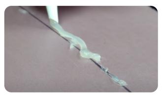
3. Put caulk over the drawn line and spread it using a putty knife [ Video 1, 21:38 ]
