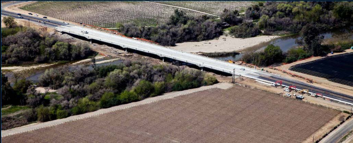
Avenue 416 Bridge over Kings River, County of Tulare, California ASCE Region 9 Structural Project of the Year, 2014 Photo Credit: Cornerstone Engineering
