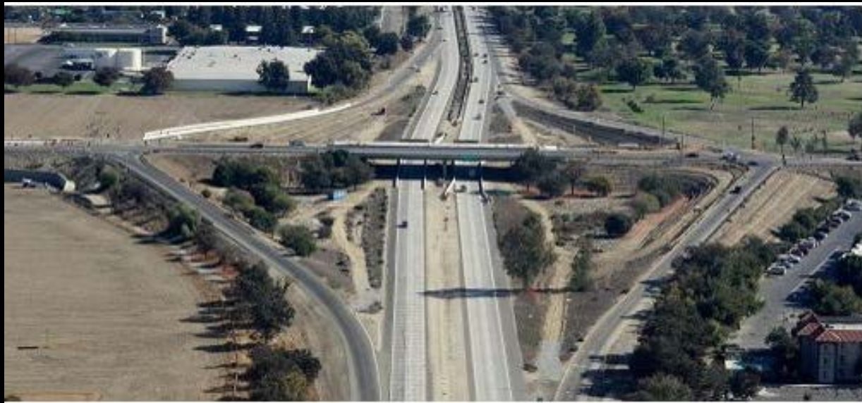
State Route 198/Plaza Drive Interchange in Visalia, California ASCE Region 9 Large Project of the Year, 2014 Photo Credit: TRC Solutions
