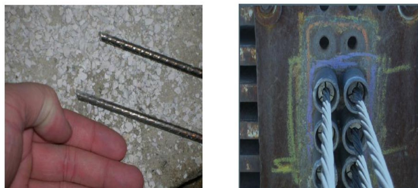
Figure 3. Single strand tendon 260ksi (left) and 7-strand tendon 270 ksi (right), (Lutch, R.H., 2009)
